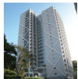
High-rise Isolated Building where Earthquake and Wind Observation are Carried out in Suzukakedai Campus
