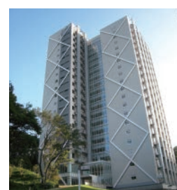
High-rise Isolated Building where Earthquake and Wind Observation are Carried out in Suzukakedai Campus
